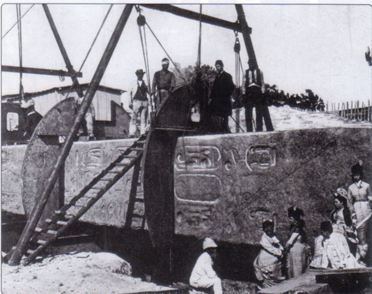
Cleopatra's Needle in Alexandria, Egypt, 1877 – showing the beginning's of Baker's cylinder being built around the obelisk. This cylinder would enable it to be transported by sea to London. Photograph courtesy Getty Images.
